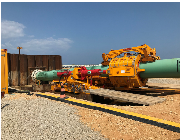
Figure 3. A.Hak 2 × 750 t Direct Pipe set in operation.
