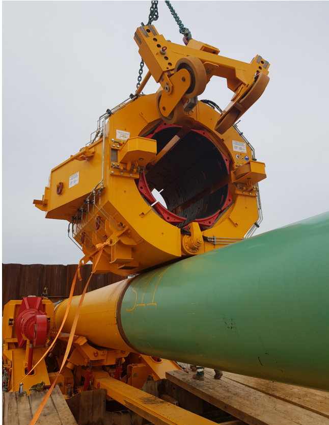
Figure 1. Installing A.Hak 56 in. clamp on thruster.
